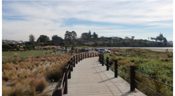
Boardwalks and viewing platforms provide beach users easy access to this popular bay while protecting the vegetation cover. Tracks along the edge of boardwalks indicate that penguins have begun using areas of the restored backdune.
