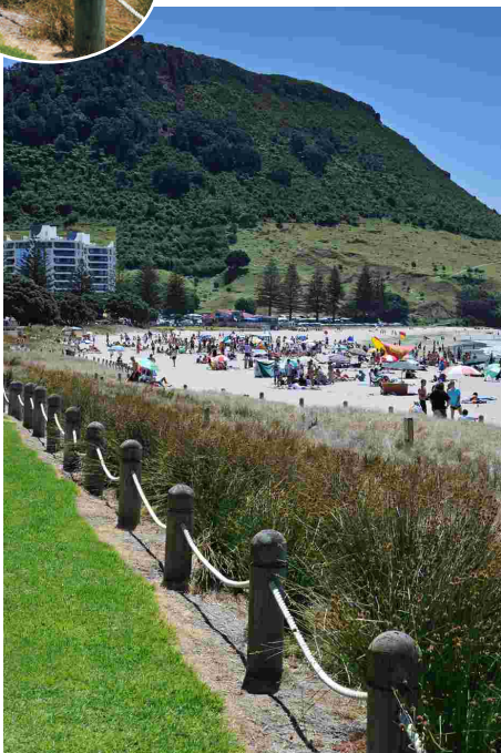
Low wooden bollards with rope are excellent for protecting dune vegetation. Bollard and rope fences are proving effective at the heavily used Mount Maunganui beach both along the landward side of the zone of sand binders (left) and along the toe of the foredune (right).
