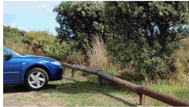
Low fixed wooden barriers placed around carparks on dunes prevent vehicles accessing dune systems.
