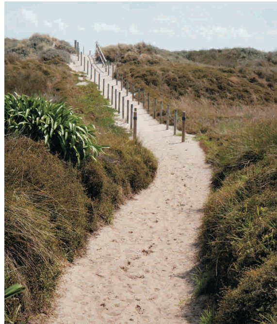
Combinations of fence types and use of vegetation as a barrier are used on many sites. A post and rope fence has been constructed on the seaward face of the foredune to protect highly vulnerable native sand binders but landward no fence is required where dense vegetation effectively defines the walking track.
