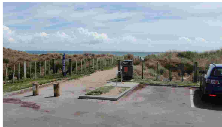
It is usually not necessary to erect a stock-proof type fence on dunes to control pedestrian traffic. Most beach users will not enter fenced areas when even the most basic fence construction is used, and especially if sufficient, well signposted accessways are provided.
