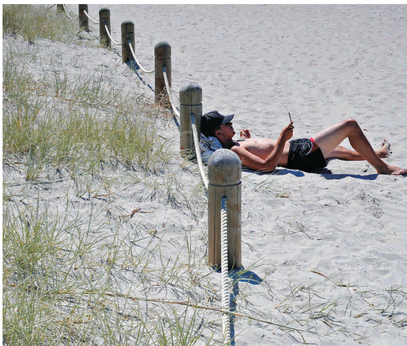
Low wooden bollards with rope are excellent for protecting dune vegetation. Bollard and rope fences are proving effective at the heavily used Mount Maunganui beach both along the landward side of the zone of sand binders (left) and along the toe of the foredune (right).
