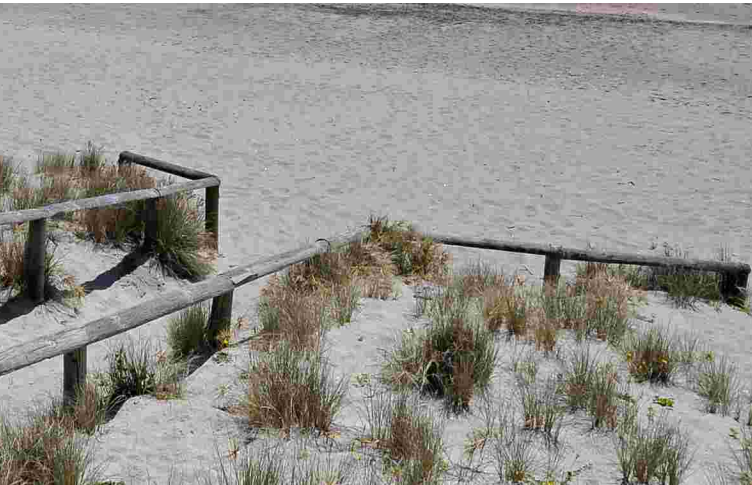
A short section of fence either side of the ends of accessway, or 'wings' may be all that is necessary to encourage pedestrians to keep to formal tracks.
