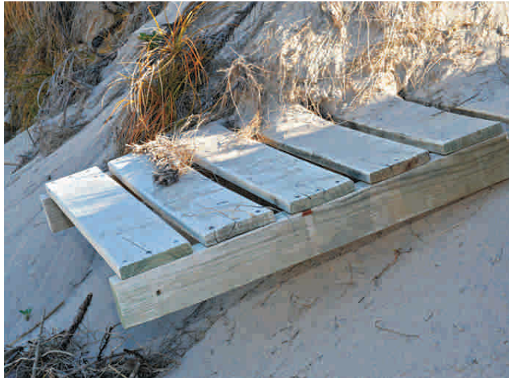
Solid wooden structures are only suitable for erecting on the more stable well vegetated landward parts of dune systems to provide access. However, ultimately most will become undermined, damaged or completely destroyed by wave action during high seas or major storms.
