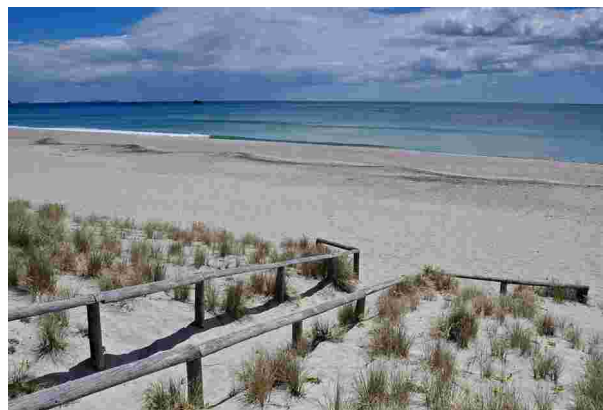
Ensure fences along accessways are placed immediately adjacent to board walks to prevent beach users creating erosion-prone bare sand tracks either side.
