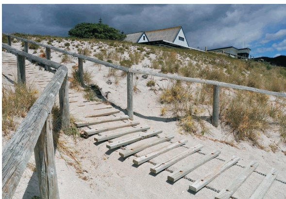
Fencing that splays outward at the toe of this foredune has caused a Y-shaped embayment along the seaward line of sand binding vegetation, even though the sand ladder continues down to near high water mark. Fences should be taken to the edge of the seaward vegetation to prevent beach users taking short cuts.
