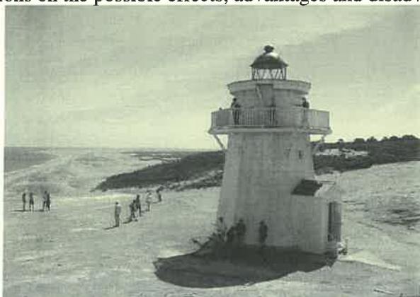
Kaipara Head lighthouse sits high on an outcrop overlooking the entrance to the Kaipara Harbour. Sand drifts had built up around and inside the building, covering most of the entrance steps on the right for many decades. It is hoped that the recent clearance of vegetation will discourage sand from accumulating at the exposed site.
