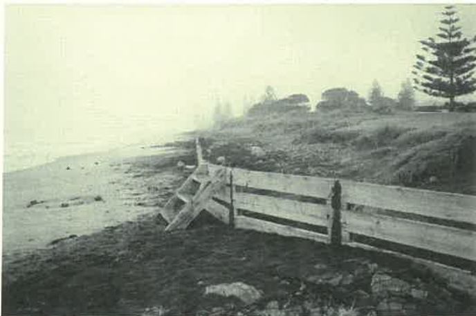
Brighton Reserve seawall before the restoration
