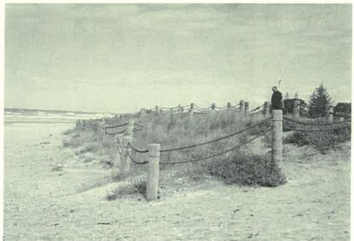
Brighton Reserve beach after restoration
