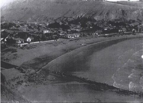
The Sumner Esplanade and rock revetment at Scarborough Beach was constructed in stages from around the early 1930s through to the early 1950s. Prior to this the beach was backed by a sand dune system. The dunes succumbed to the early
