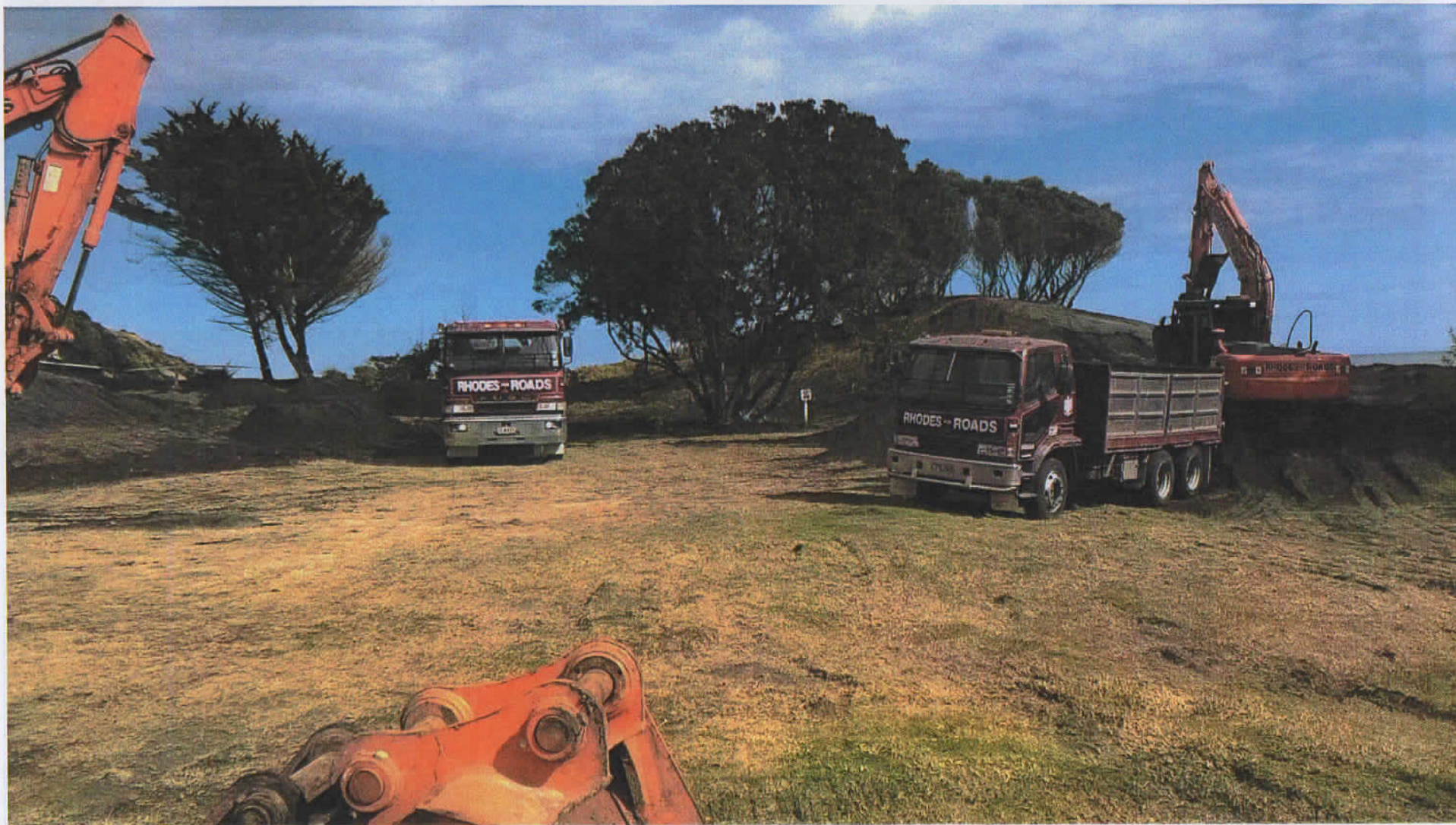
Redistribution of sand to create new backdune area for planting.
