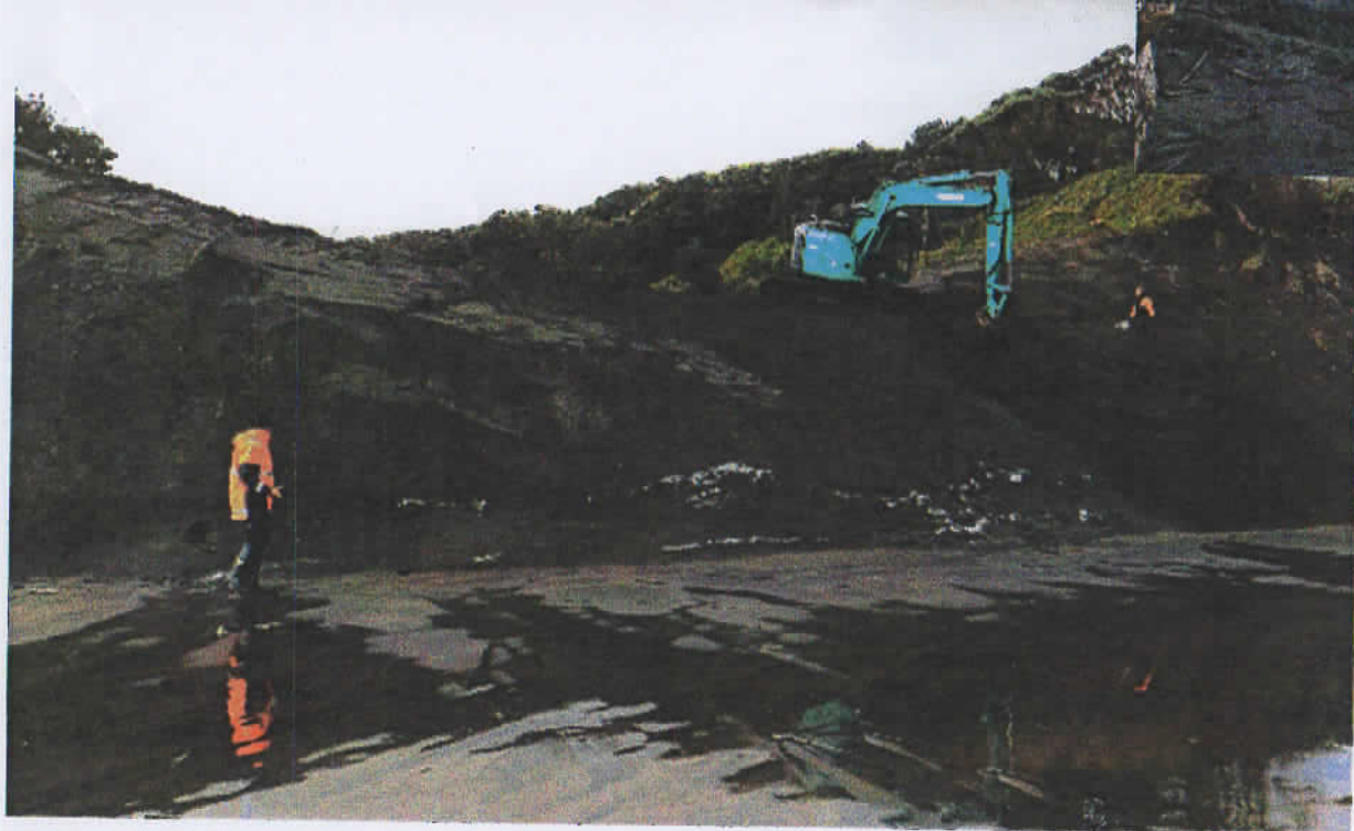
Area B reshaping/lowering.
