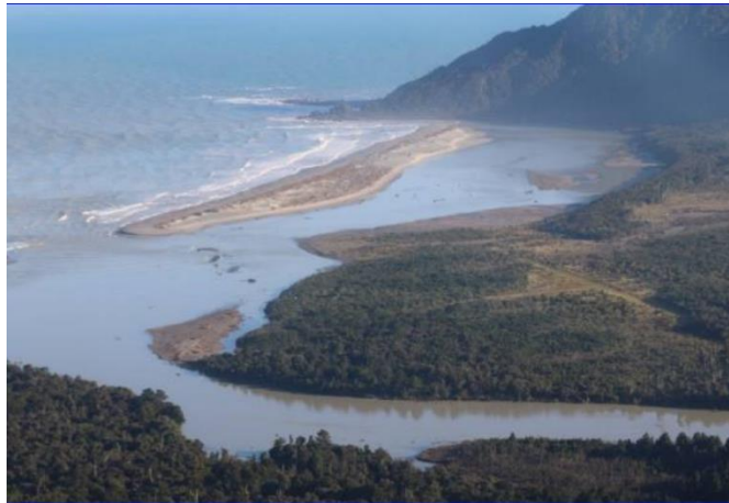
February's floods have changed the landscape
