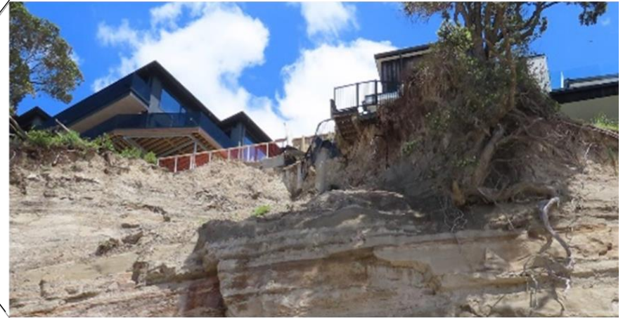
A) Location of the wedge failure with its associated vertical jointed surface/failure plane (black dashed lines). B) Failure of sandstone bedding plane C) Talus formed due to the accumulation of the debris supplied by the two failures above. D) Collapse of weathered soil at the cliff top has exposed the Pōhutukawa tree root system and foundations of the properties. A properties' deck can be seen hanging mid-air.
